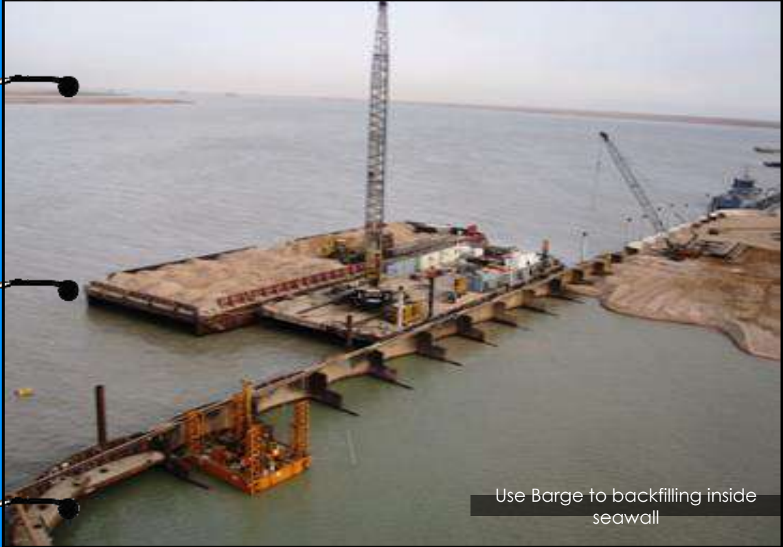
Concrete Road for seawall Um Qasr
