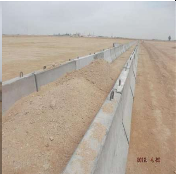
Twalls Erection around IPF
