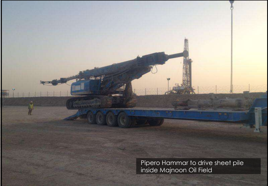
Construction of Manjoun Jetty Pits
