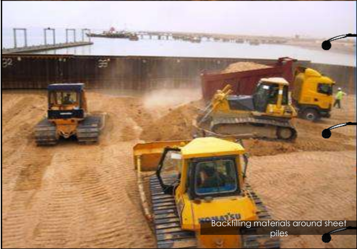
Supply of backfilling materials around 300,000 m 3
